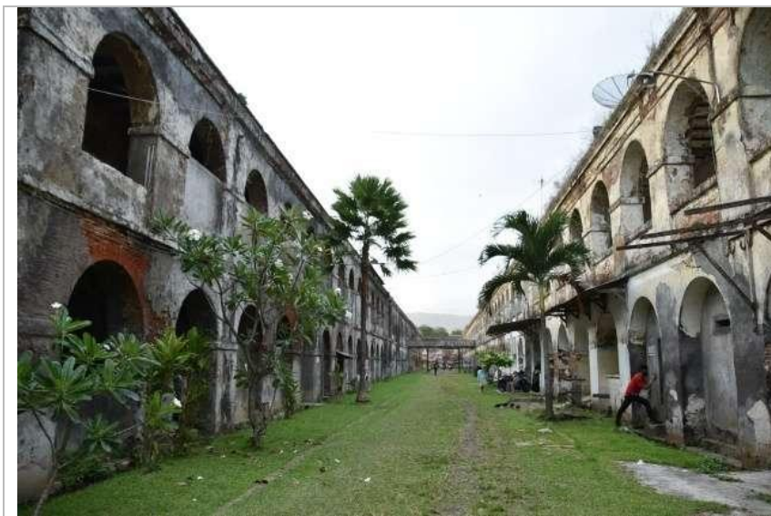
Figure 6. The condition of Willem I Fort before its revitalization. Source: jatengprov.go.id (2020)
