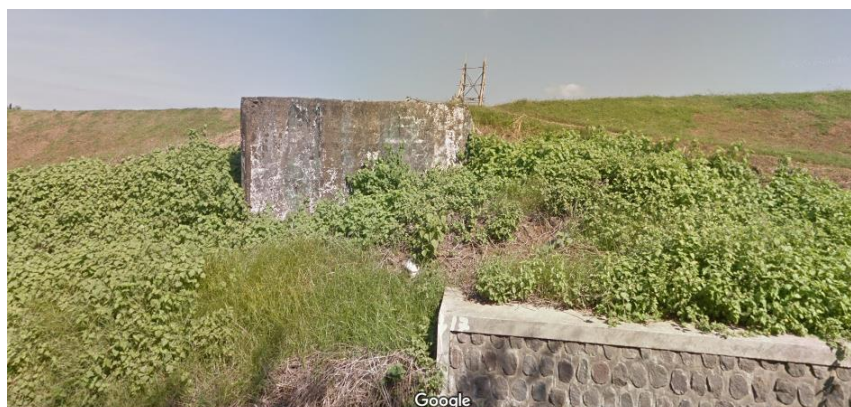
Figure 2 Pillbox Kedunglangkap from the east
